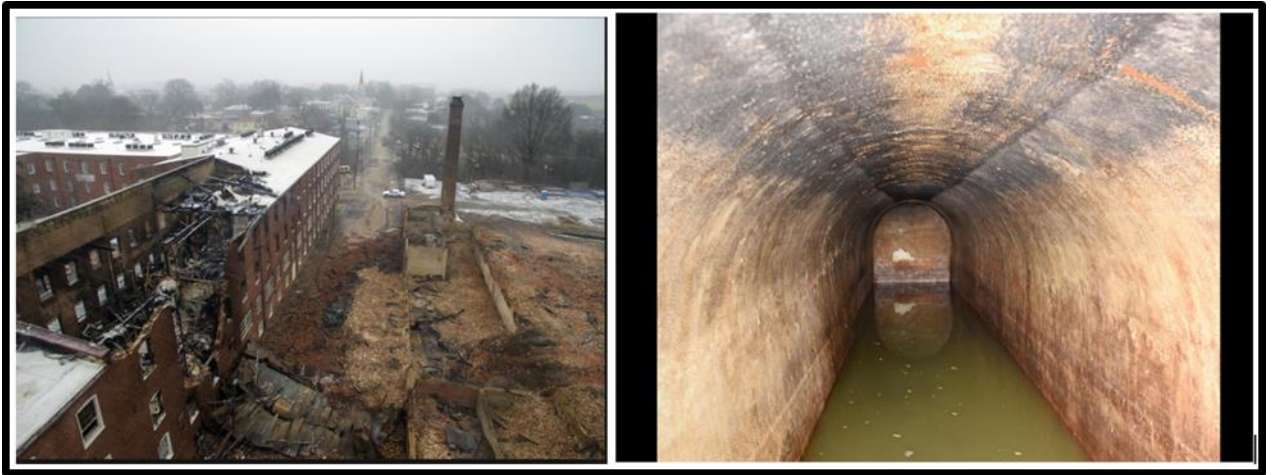
Figure 5. Drone image of factory fire in 2018 (left) and uncovered conduit discovered by public works while cleaning up the site. These images are available through the federal Freedom of Information Act on the city website.
