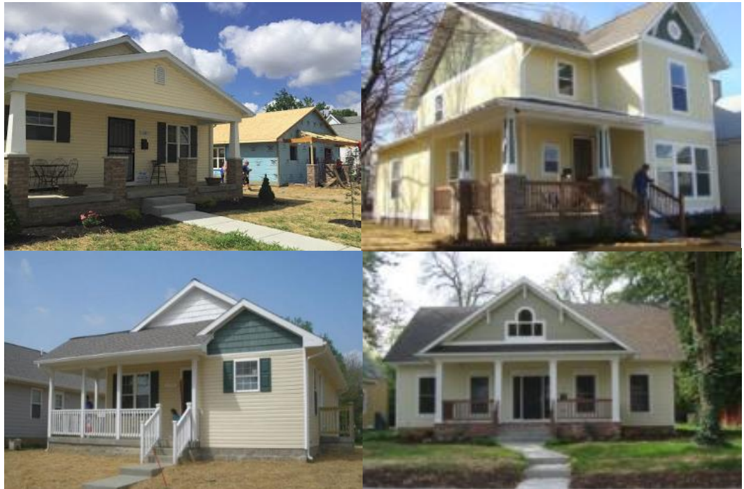
Figure 11. New houses built by local nonprofit developers in the Promise Zone.
