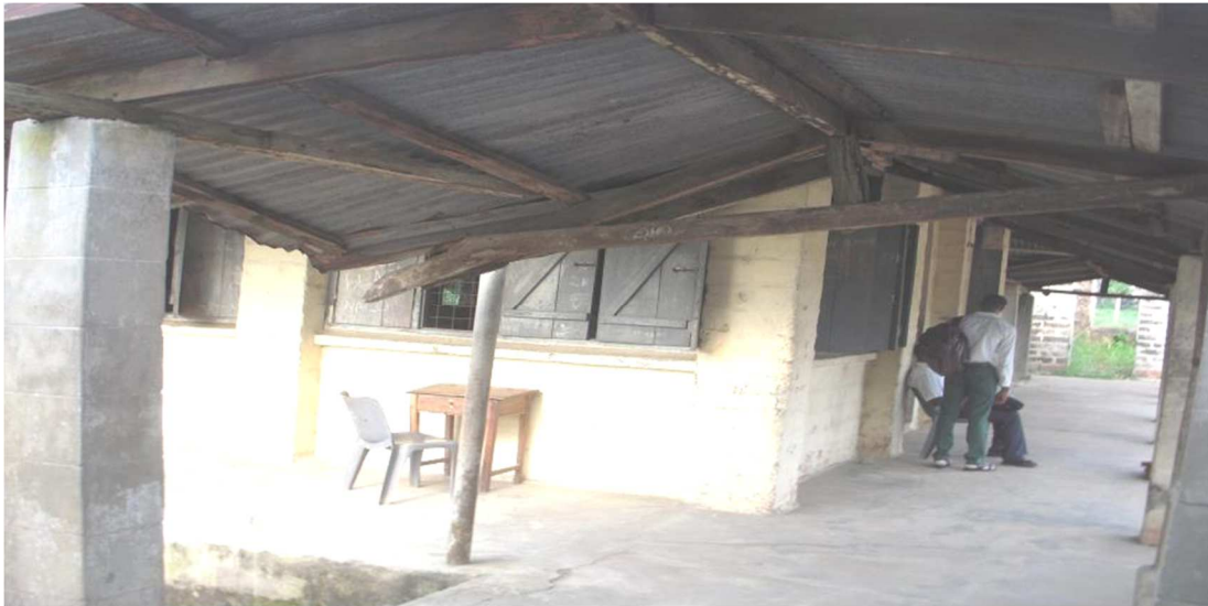
Figure 5. Picture of the roof at Shahana Secondary School
