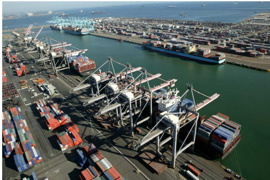
Figure 1. View of a section of the port, showing piers for ship mooring and cargo transfer.
