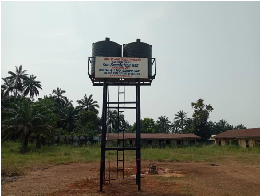
Figure 4. Picture of a noncommercial borehole.
