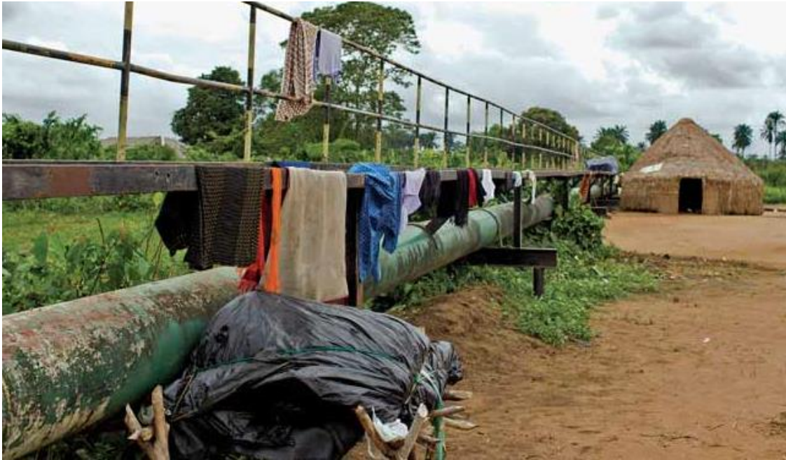
Figure 9. A traditional house made from combustible materials adjacent to a pipe line (Ebubu, Obolo-Eleme LGA) Source: UNEP Assessment, (2011).
