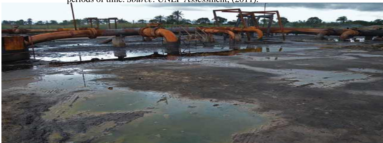
Figure 8. A view of a decommissioned and abandoned flow station in K-Dere, Ghokana LGA. Source: UNEP Assessment, (2011).
